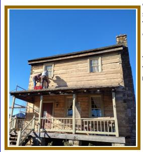
and a few other logs are being replaced. The round Neel cabin logs, typical of earliest homes, have been shaved flat to eliminate the spaces where water and insects have long collected. The buildings were treated for insects and Tanner will apply materials to strengthen and protect the wood for the future. And finally fresh chinking will keep out the birds, bugs and elements.
